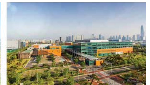
The Second Manufacturing Plant 90,000 liters (6 lines x 15,000 liters)
