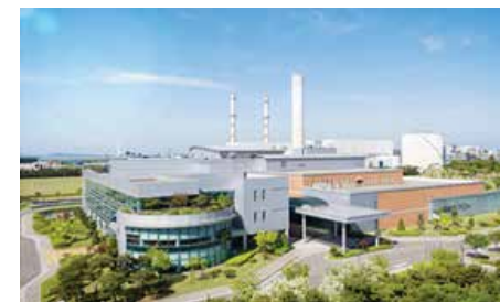
The First Manufacturing Plant 50,000 liters (4 lines x 12,500 liters)
